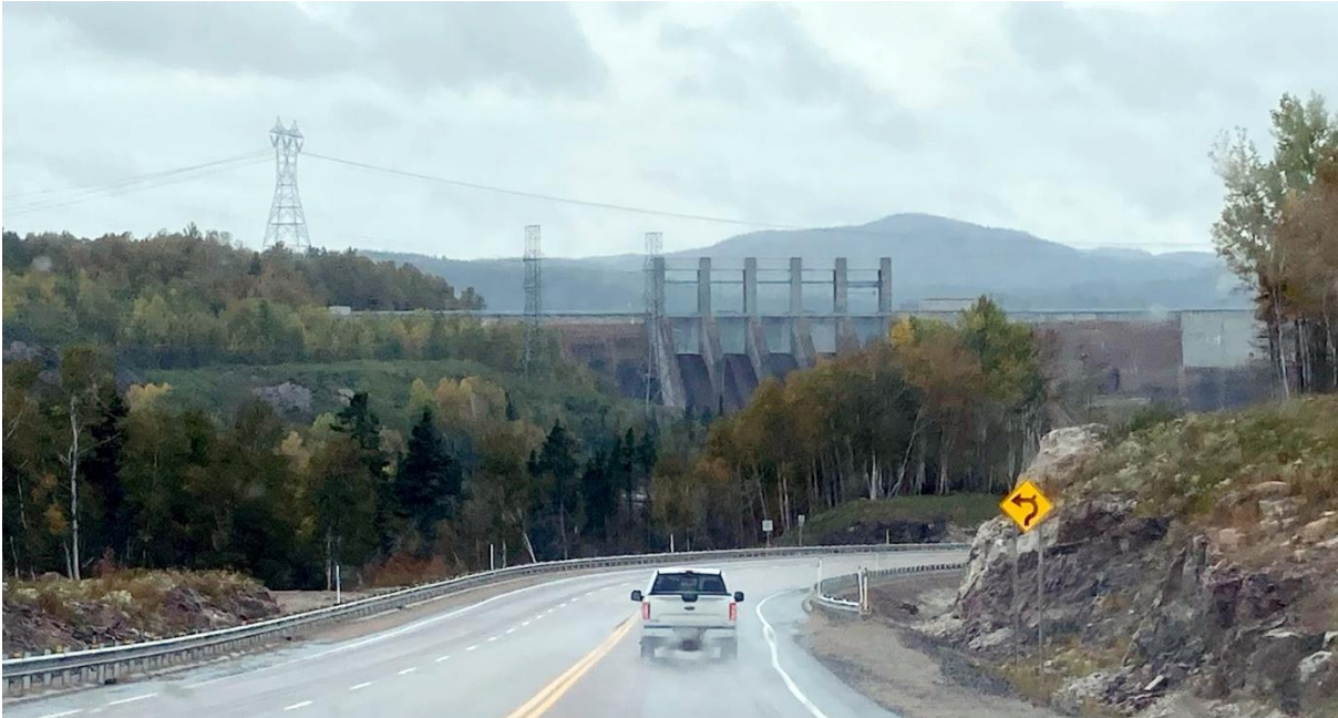
View of a dam in the Pessamit reserve, 2022 © Camille Ducroquet/Amnesty International
